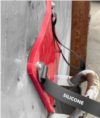
The patch perfectly conforms to the irregularities of the damaged surface
